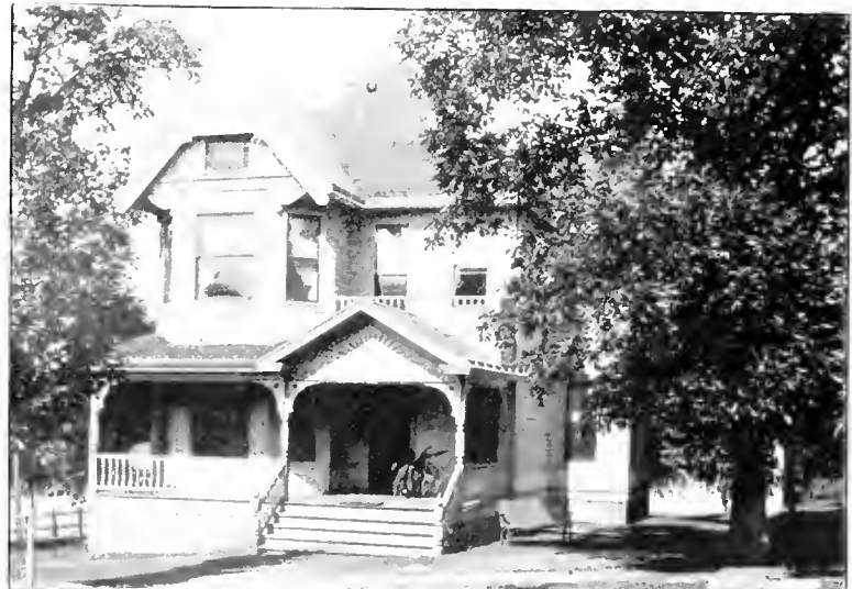
RESIDENCE OF S. A. PRATER, North 7th Street.
